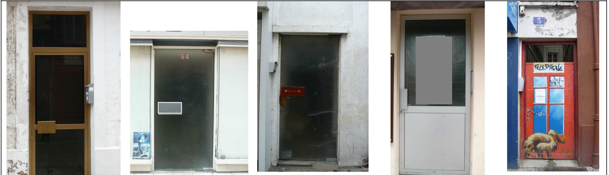
REPLACEMENT DES PORTES D'IMMEUBLES PAR DES MODELES EN TOTALE INCOHERENCE AVEC LA TYPOLOGIE ARCHITECTURALE ET LA QUALITE DES CONSTRUCTIONS DU CENTRE ANCIEN (MATÉRIAU, MODÈLE, POSITION)
